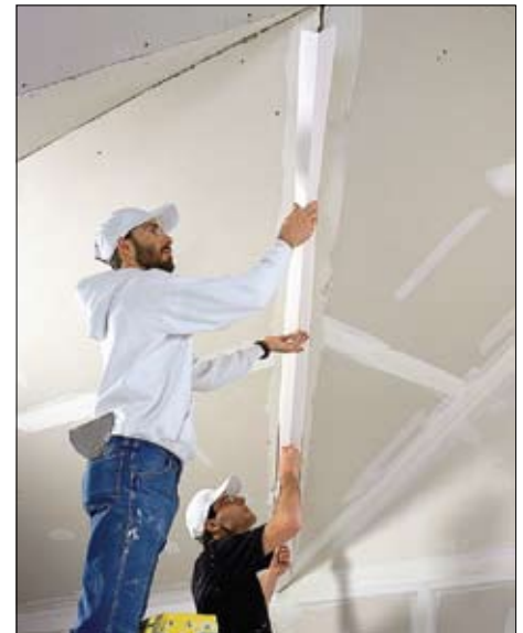
NO-COAT ULTRAFLEX Application
