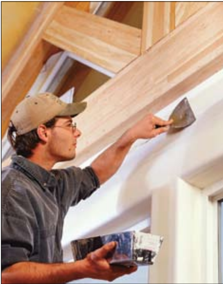
NO-COAT L Trim Install
